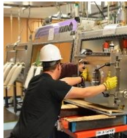
New Backfill Station Installation
