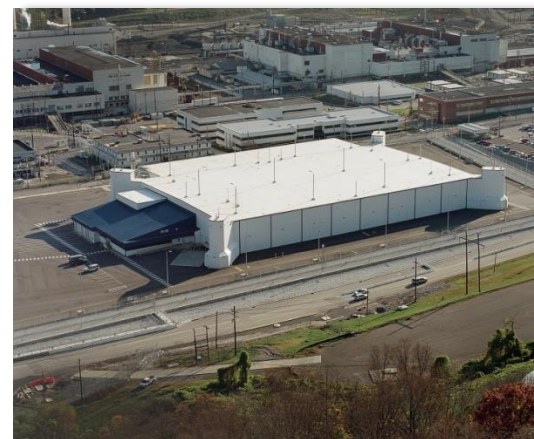
Aerial View – Highly Enriched Uranium Materials Facility 3
